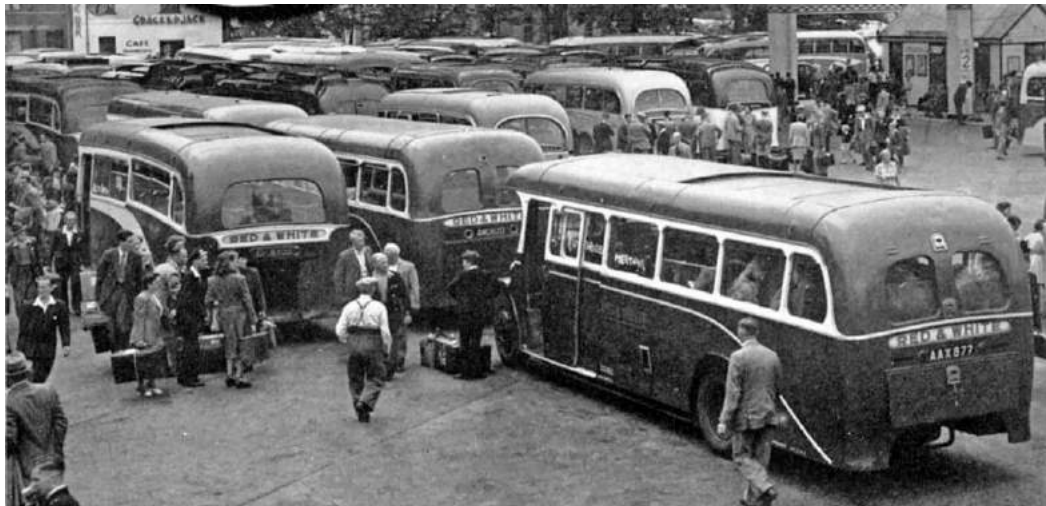
Duple-bodied Albion Valkyries at Cheltenham Coach Station. 1936 Valkyrie SpPW69 AAX 877 (277) foreground and 1936 Valkyrie SpPV141 AWO 620 (307) in front. The coaches have had their roof-mounted luggage carriers removed but still have the rear steps used by the driver to reach the roof. On the left is a 1938-39 Valkyrie CX13. ( Red & White Services 1919-1949 )
