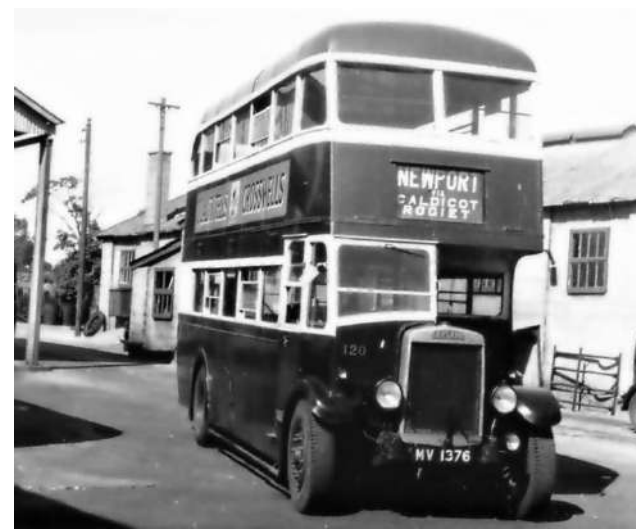
Front and rear views of Leyland Titan TD2 MV 1376 after rebodding with a second-hand East Lancs H30/26R body.
